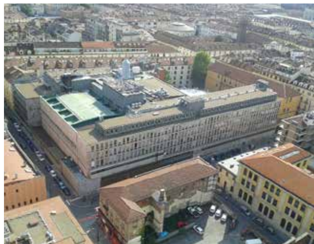
Turin Production Centre - Via Verdi
