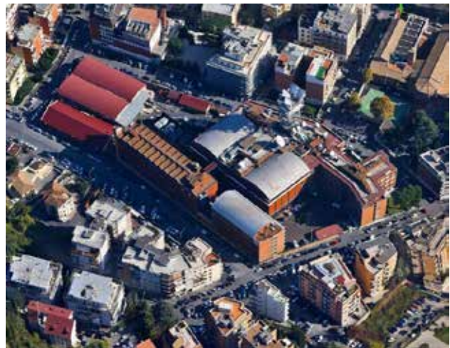
Rome Production Centre - Via Teulada
