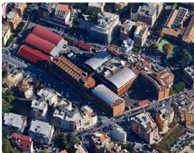
Rome Production Centre - Via Teulada
