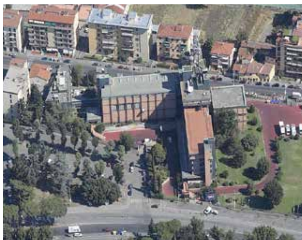
Rai Regional Headquarters in Florence - Via Bernabei
